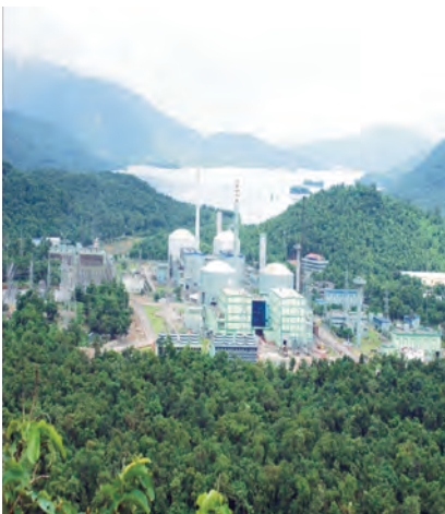
Fig. 4. Nuclear Power plants at Kaiga in thick western ghat forest of Karnataka
